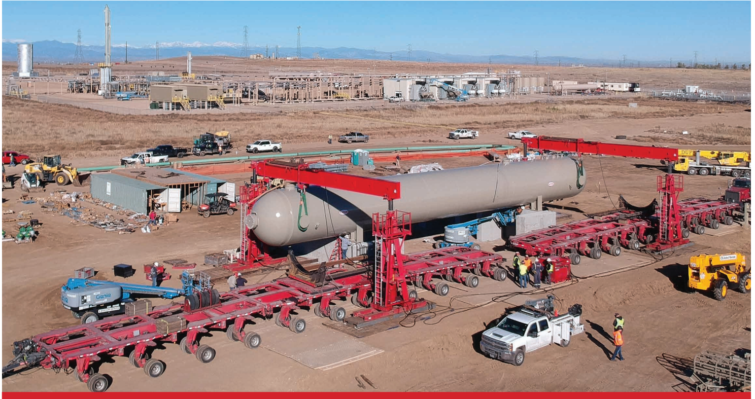
Industrial Gas Processing: Barnhart used a dual-lane over-the-road trailer and 500-ton gantries to deliver and set a 634,000-pound natural gas sludge catcher.
