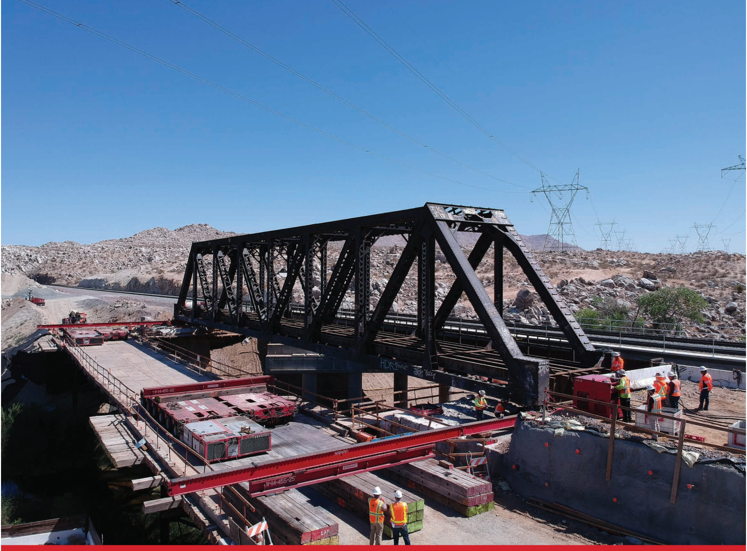
Heavy Civil: The team uses SPMT and jack and slide to move an 800,000-pound bridge.
