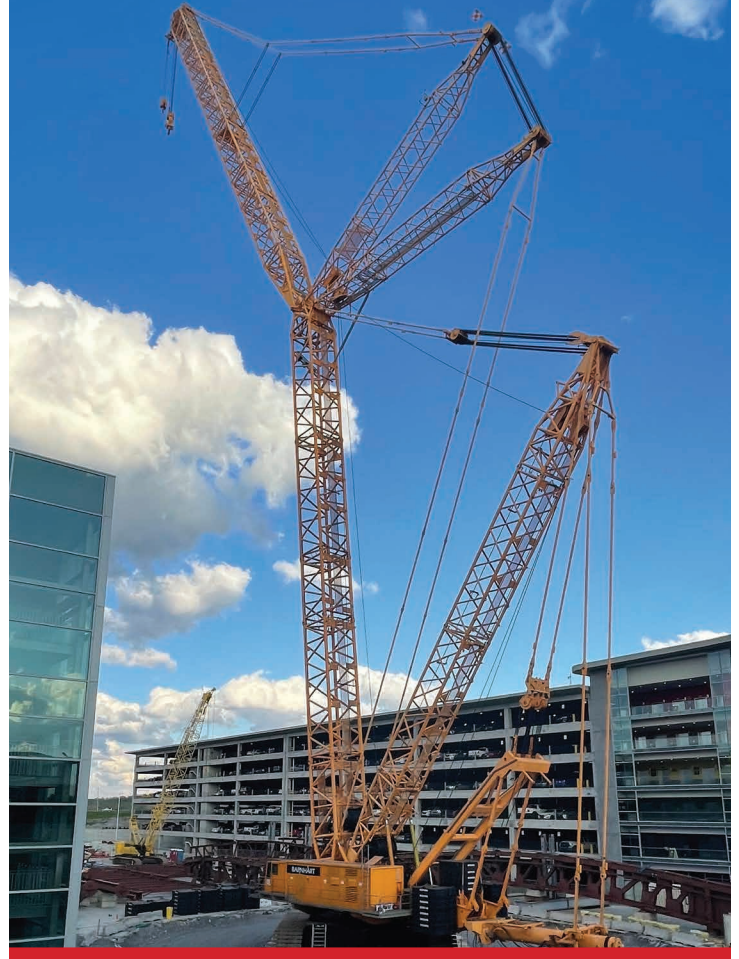
The CC8800 helps with construction at the Nashville airport lifting 180-kip truss sections at a 328-foot radius.
