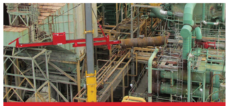
Refining: Barnhart uses its MOCCS cantilevering system to streamline heat exchanger replacements in a local refinery.
