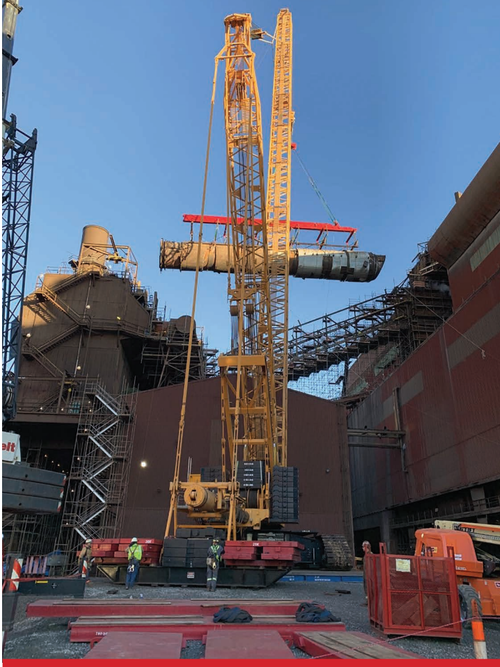
The CC8800 in action at a steel mill with customized rigging that provided horizontal rotation in the air.
